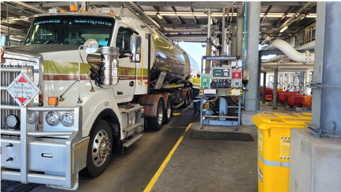
2. Truck Loading Gantry showing control panel and spill kit
