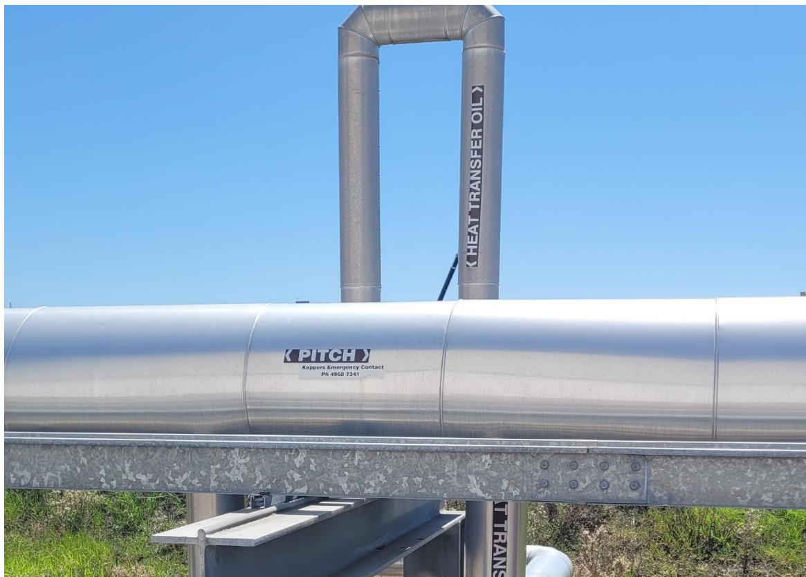
14. Example signage on the pipeline to Mayfield 7 (M7) Berth including emergency contact details
