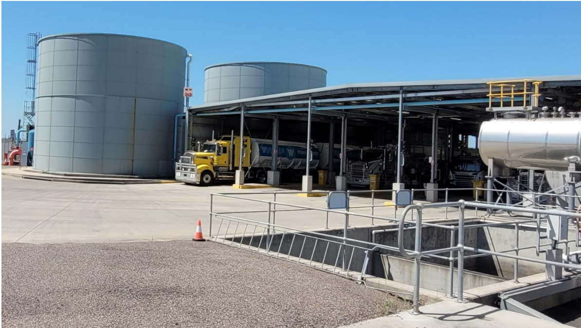
1. Truck Loading Gantry (Looking South) with First Flush Stormwater Pit in foreground
