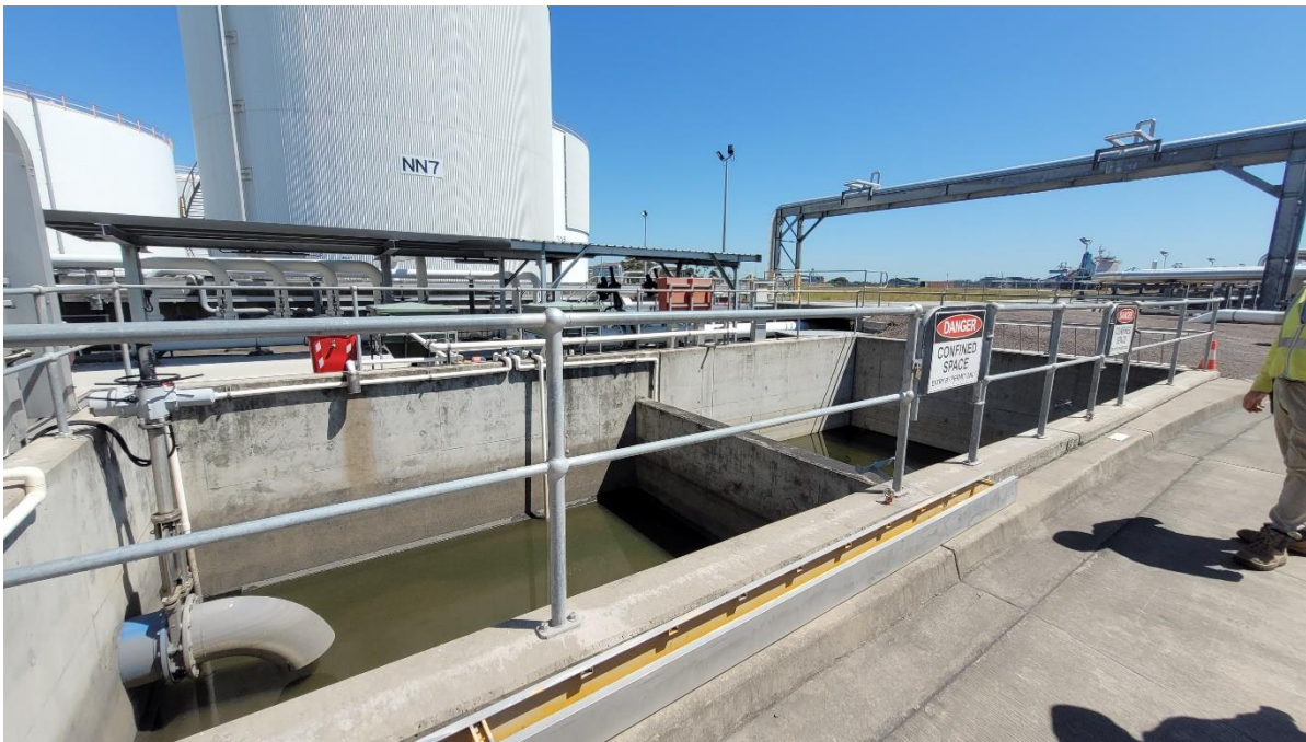
7. First Flush Stormwater Pit
