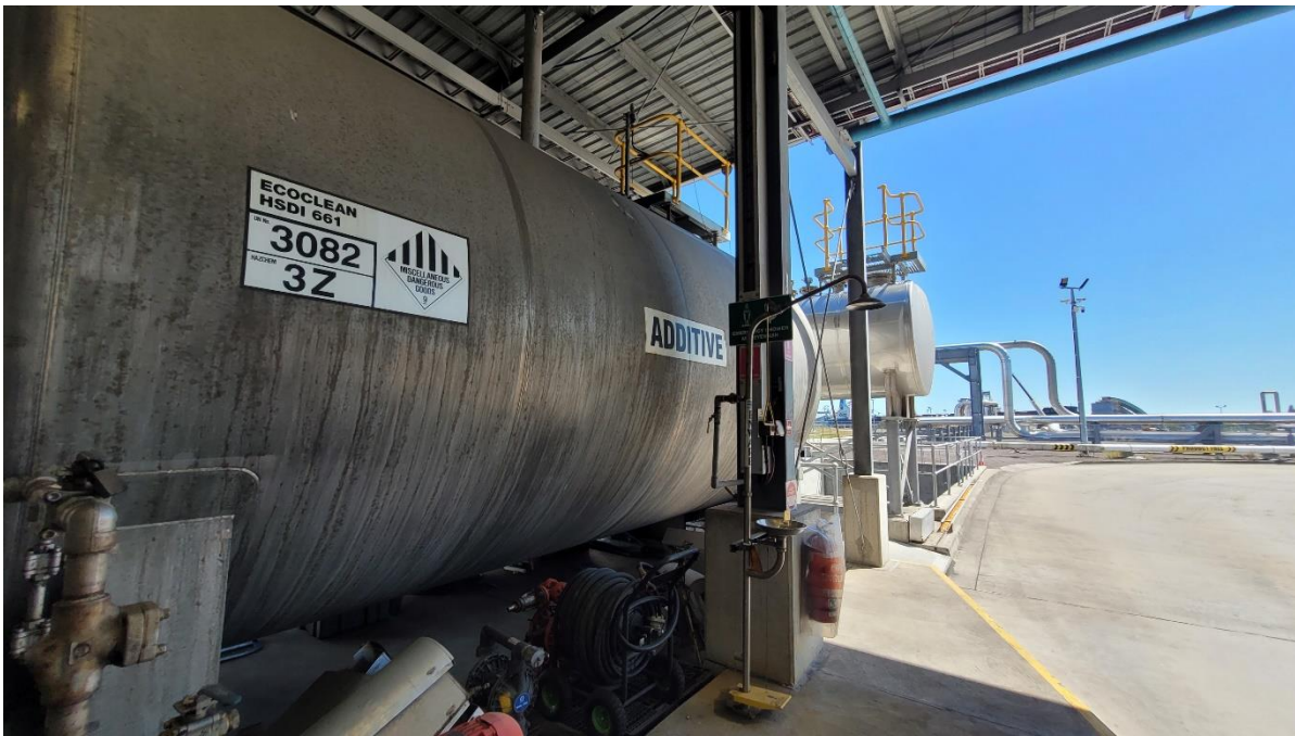
5. Truck Loading Gantry Additive Tank (1)
