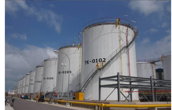
Stolthaven Singapore Gas sphere and Bulk chemical tanks
